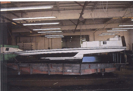
This is the deck being removed from its mold. The window accent color and the non-skid surfaces are molded in. The deck liners have already been bonded in place.
